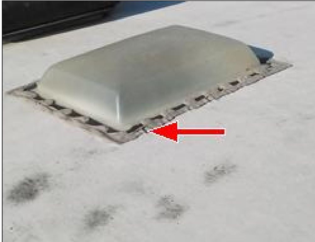
Kitchen Skylight center of trailer
