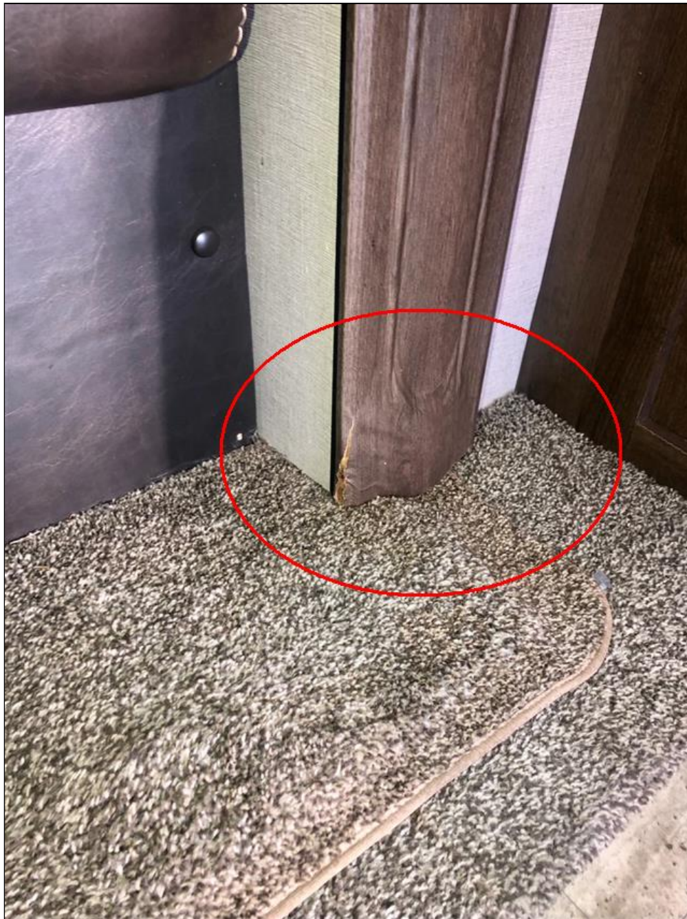
Trim work right lower side of slideout
