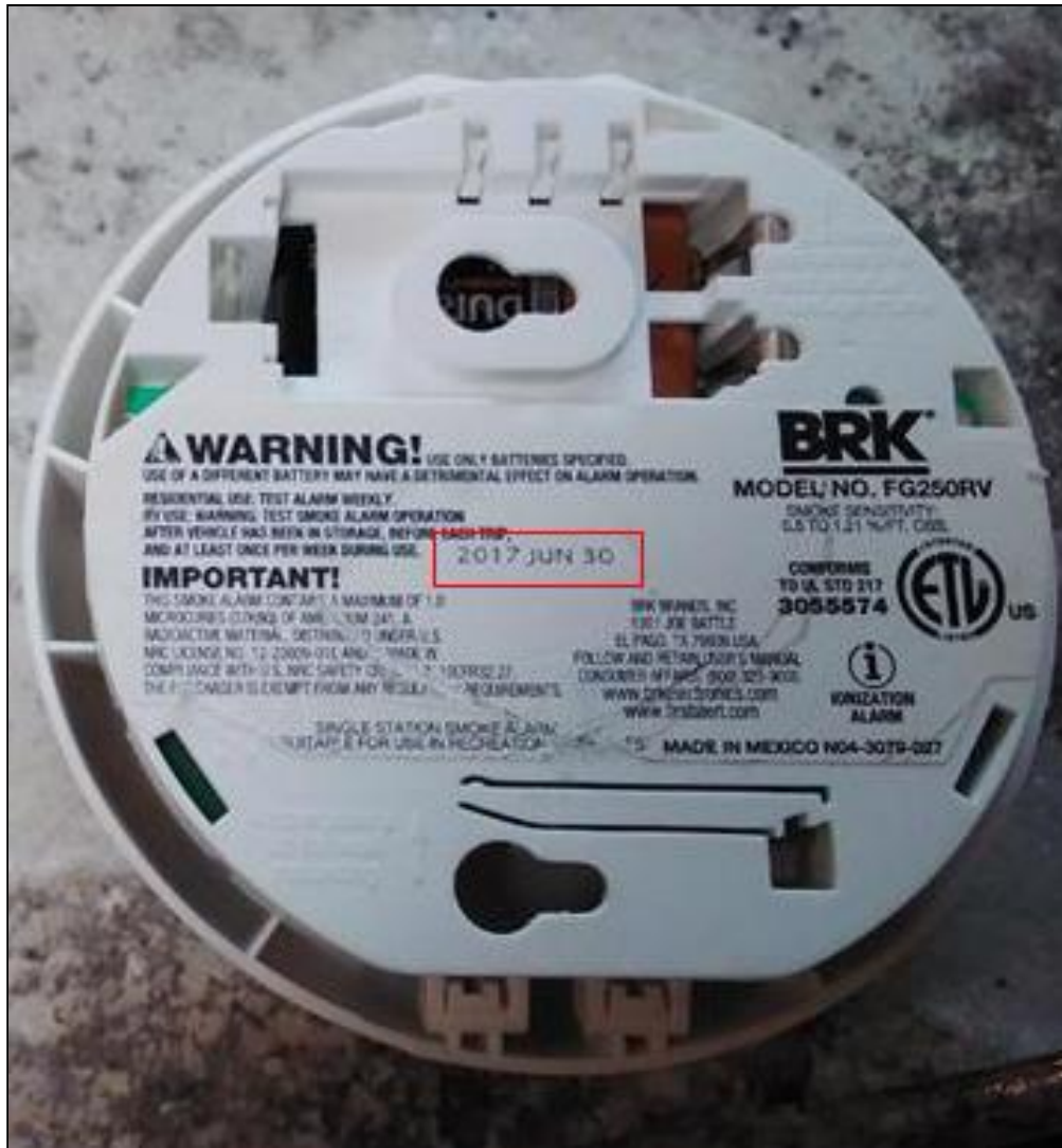
Smoke detector date
