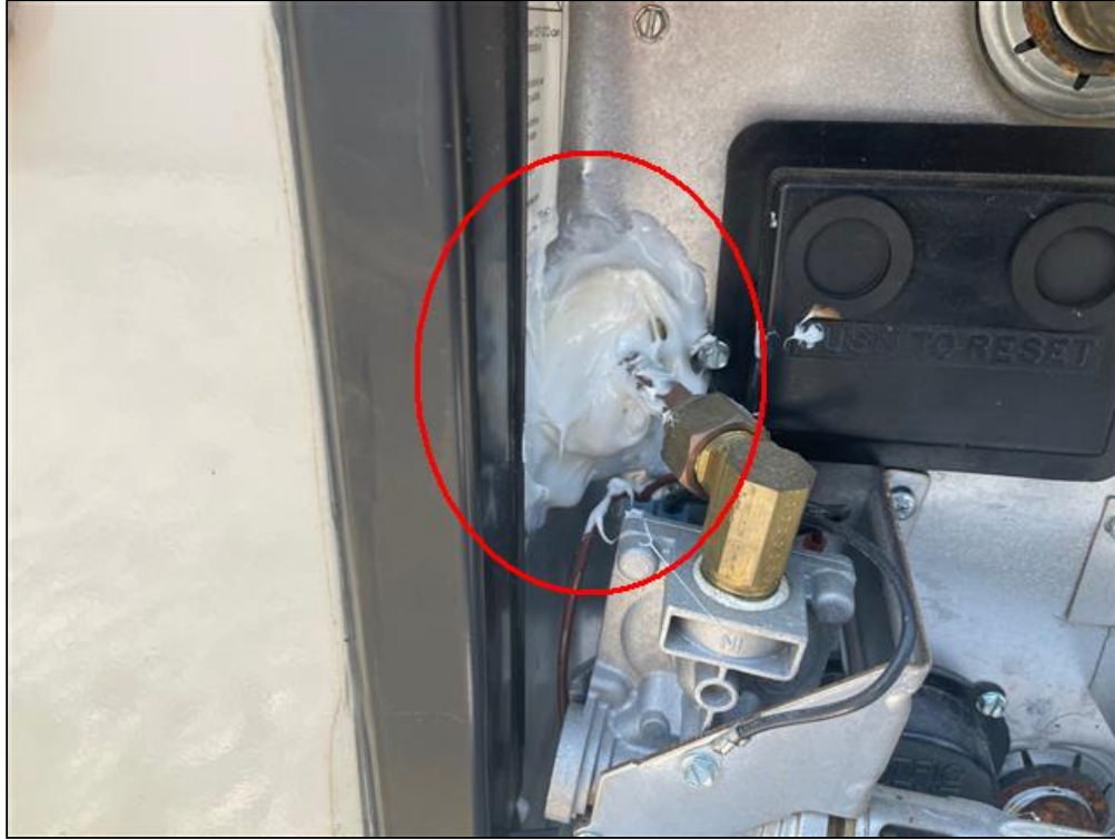
Seal around gas fitting
