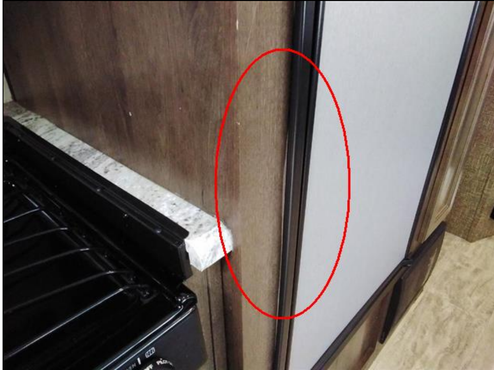
Left lower side refrigerator door frame
