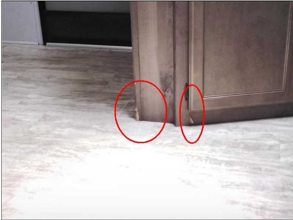
Left lower side of kitchen sink cabinet
