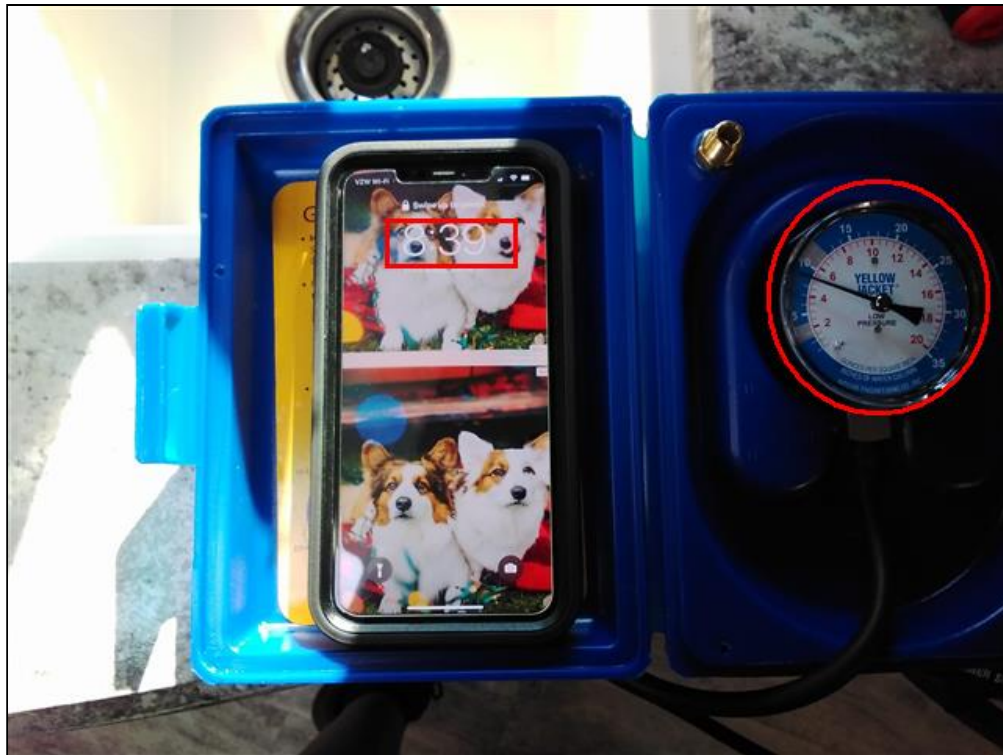
Completion of Propane Leak Test
