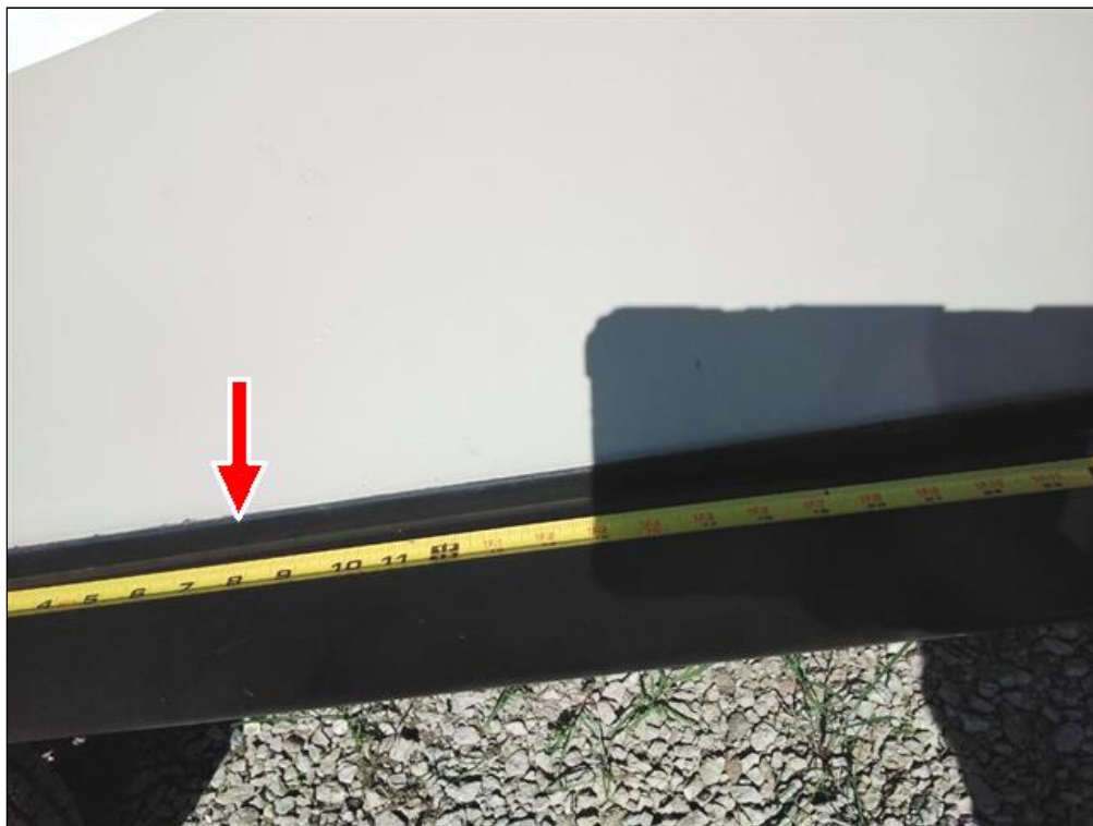
curbside behind door 1
