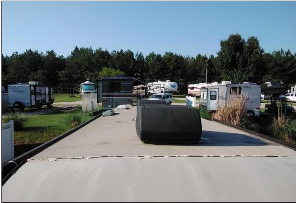
Roof Front to Back
